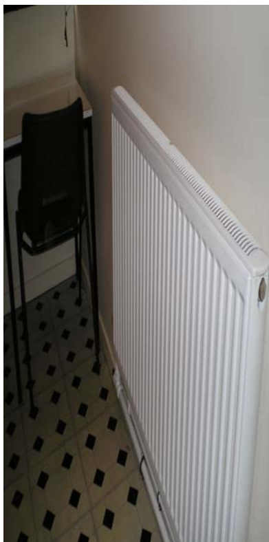
Swan House Property with new radiator installed
